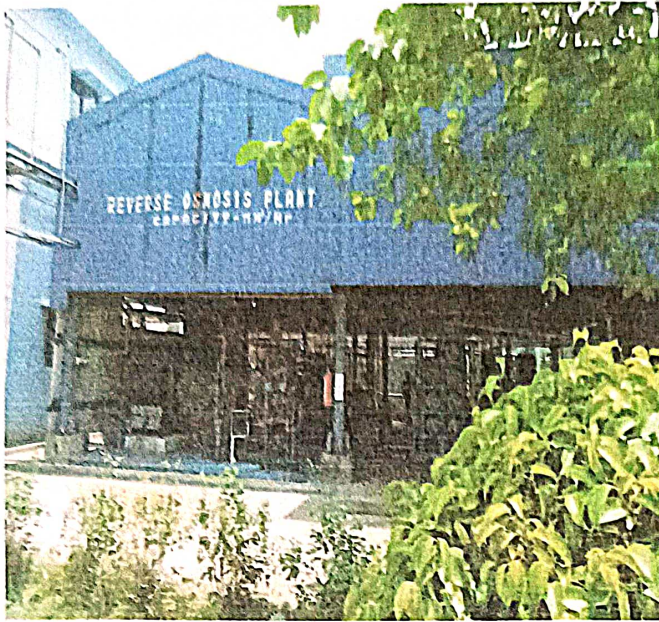
Annexure I – Picture of ETP
